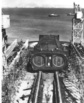
A section of the Transbay Tube being lowered into San Francisco Bay.
