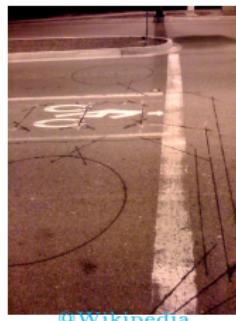
magnetic loop detectors, video recordings, floating car data, etc
